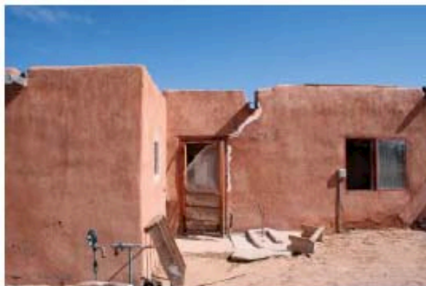
2. Exterior view of partial south elevation
