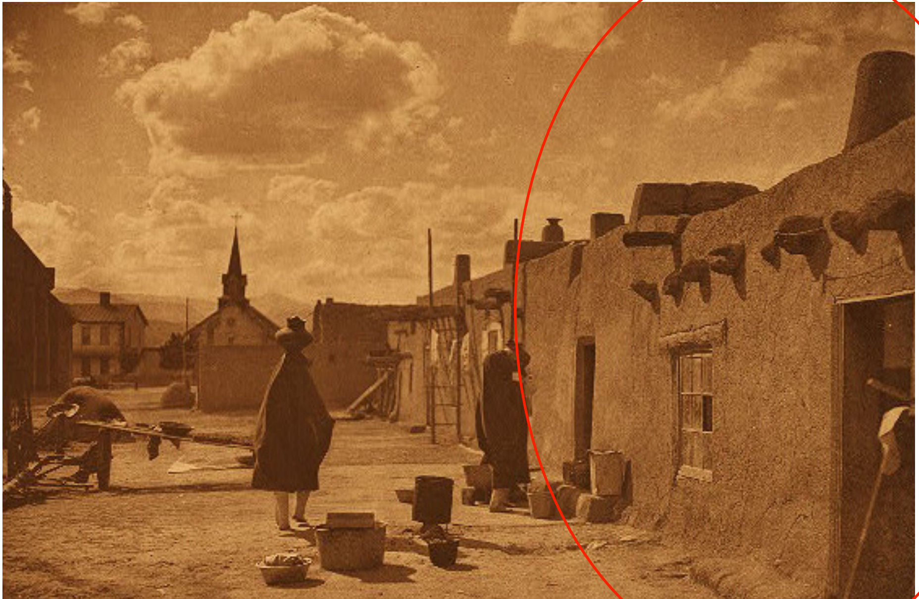
OOHPI Fig. 10-03. View looking west, Photograph by Edward Curtis, 1905
